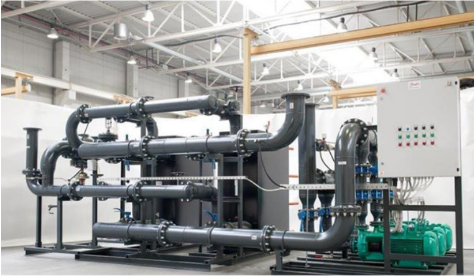
Figure 26. Typical ETS installation (source: Danfoss)
